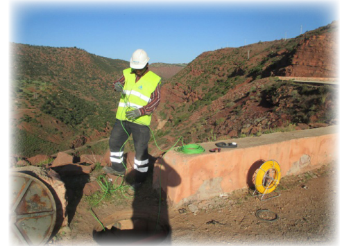
Installing digital cable for the seismic monitoring system.
