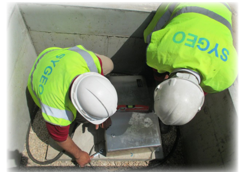
SYGEO engineers installing the seismic station.
