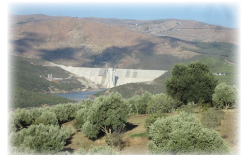
Wadi Martil Dam includes a concrete face fill dam on Wadi Mohjerat, and an earth fill secondary dam.
